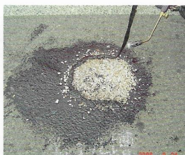
patching small pit slot
