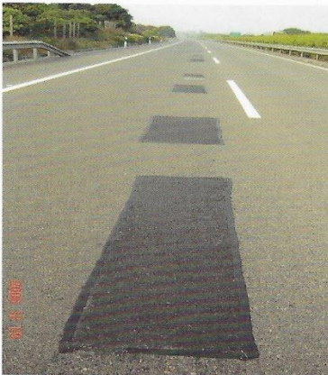
Pot holes mending and waterproof of weak seam
